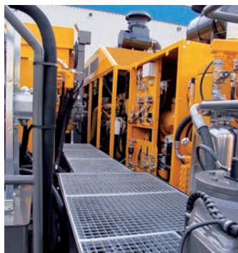
Central maintenance walk
